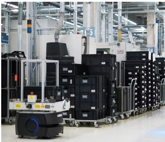
State-of-the-art intralogistics: SIMATIC RTLS (real-time locating system) gateways and SCALANCE IWLAN access points in the electronics production at Siemens in Fuerth are efficiently supplied with data and power via SCALANCE X PoE switches.
