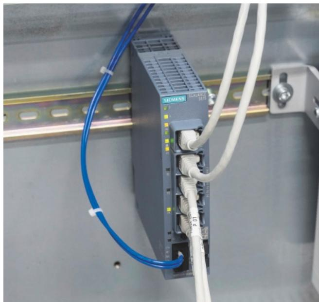
The stations of the production line are connected to the ports of the SCALANCE S615.
