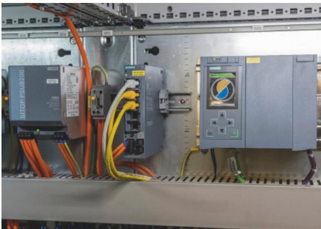
The SCALANCE S615 security appliance, the SIMATIC S7-1500 controller and the SITOP PSU8200 power supply are components installed in the control cabinet at Festo.
