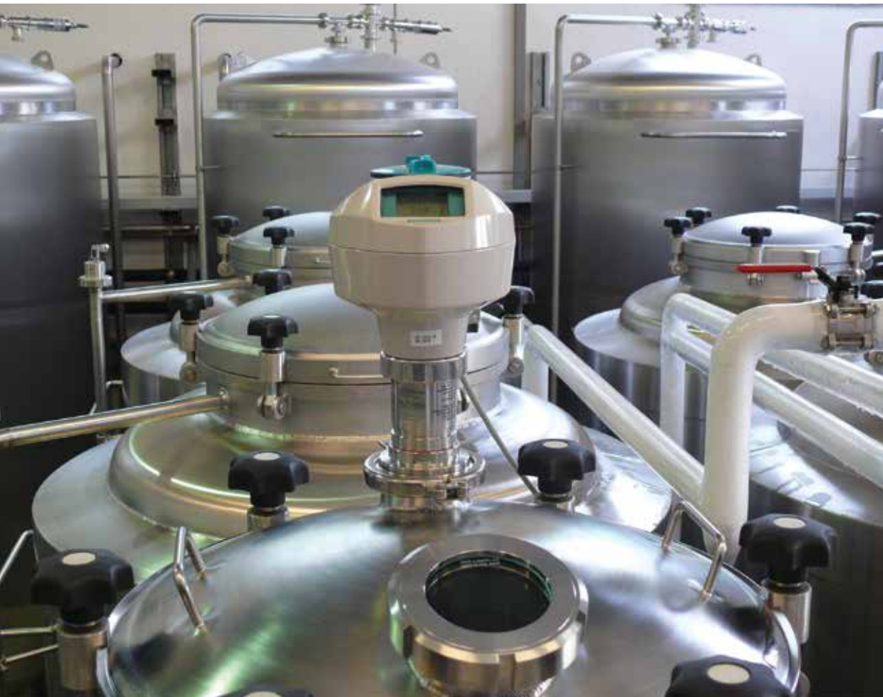
Installing the SITRANS LR250 was easy, and the facility now has reliable, high-performance continuous level measurements on their process vessels
