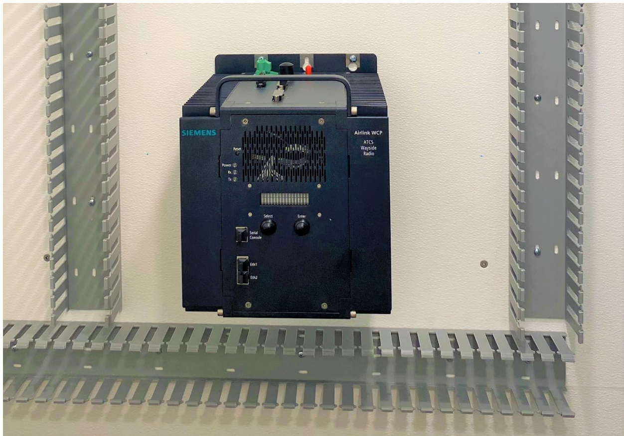
Figure 4-6 Typical Airlink WCP Wall Installation – Front View
