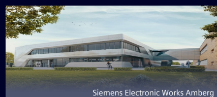
Siemens Electronic Works Amberg
