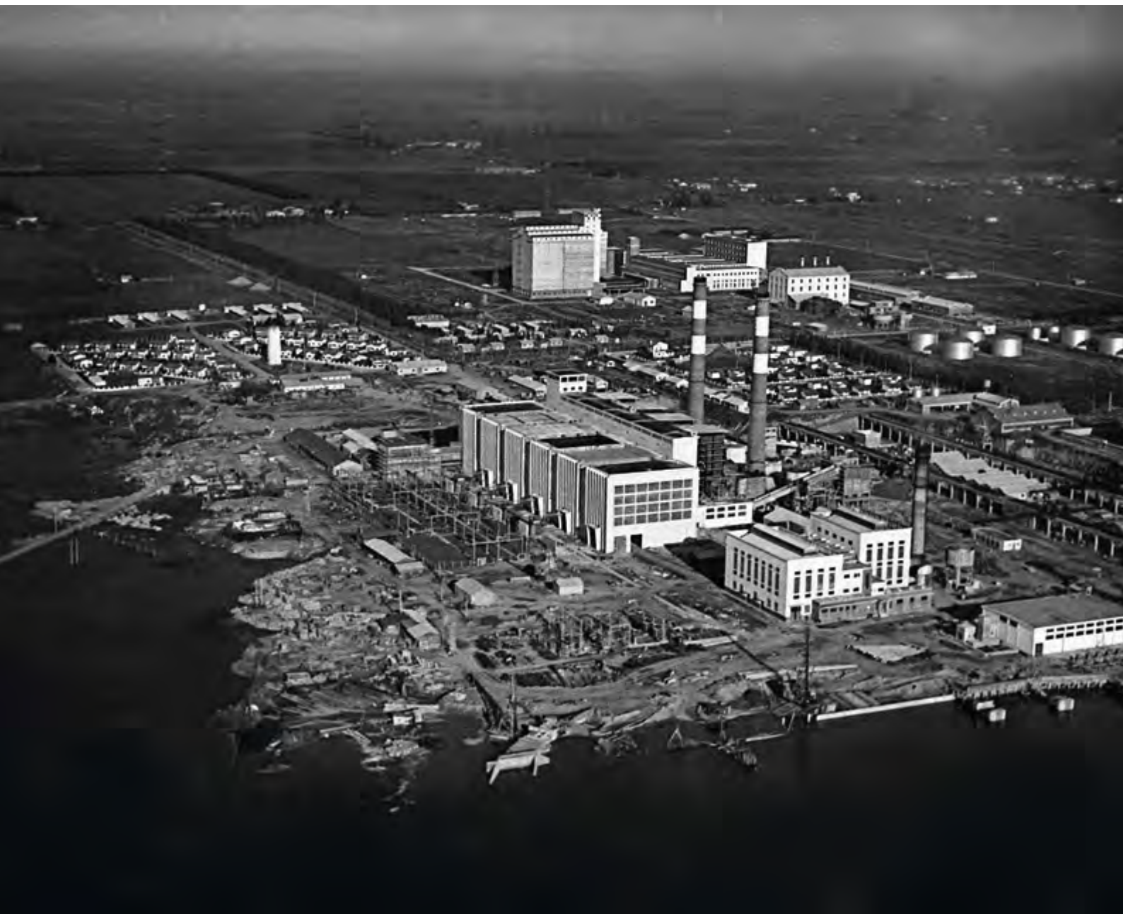
Aerial photo of the San Nicolás power plant in Argentina, 1956
