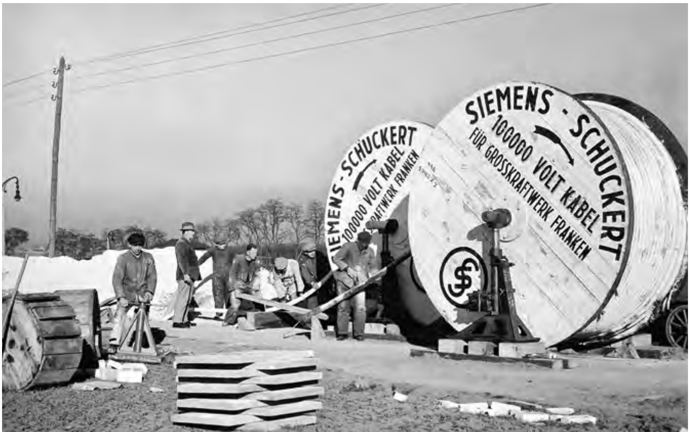
Laying a 100-kV oil-filled cable in Nuremberg, 1931
