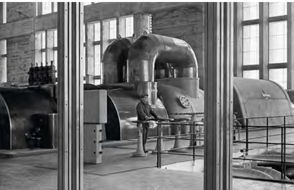
Machine room in the San Nicolás power plant in Argentina, 1956
