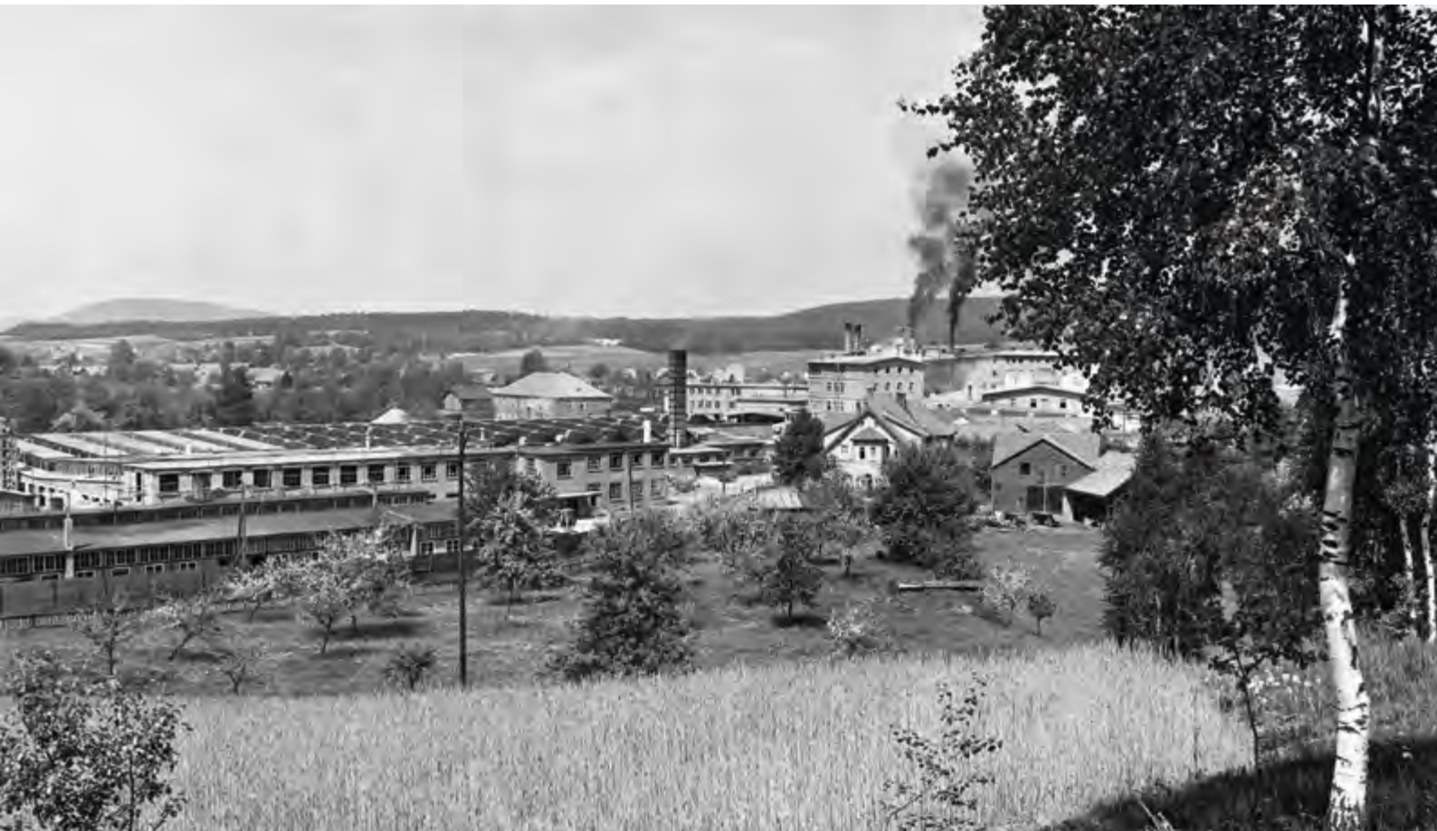
Relocation plant porcelain factory Neuhaus, 1941
