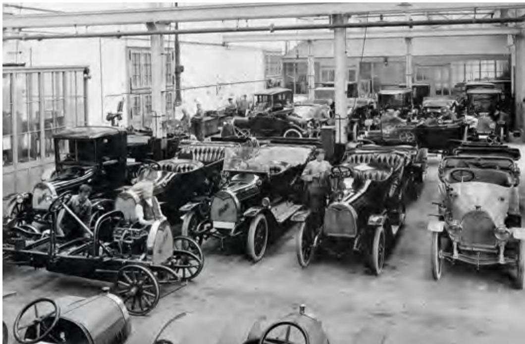
Protos cars being built at the Berlin automotive plant, 1913
