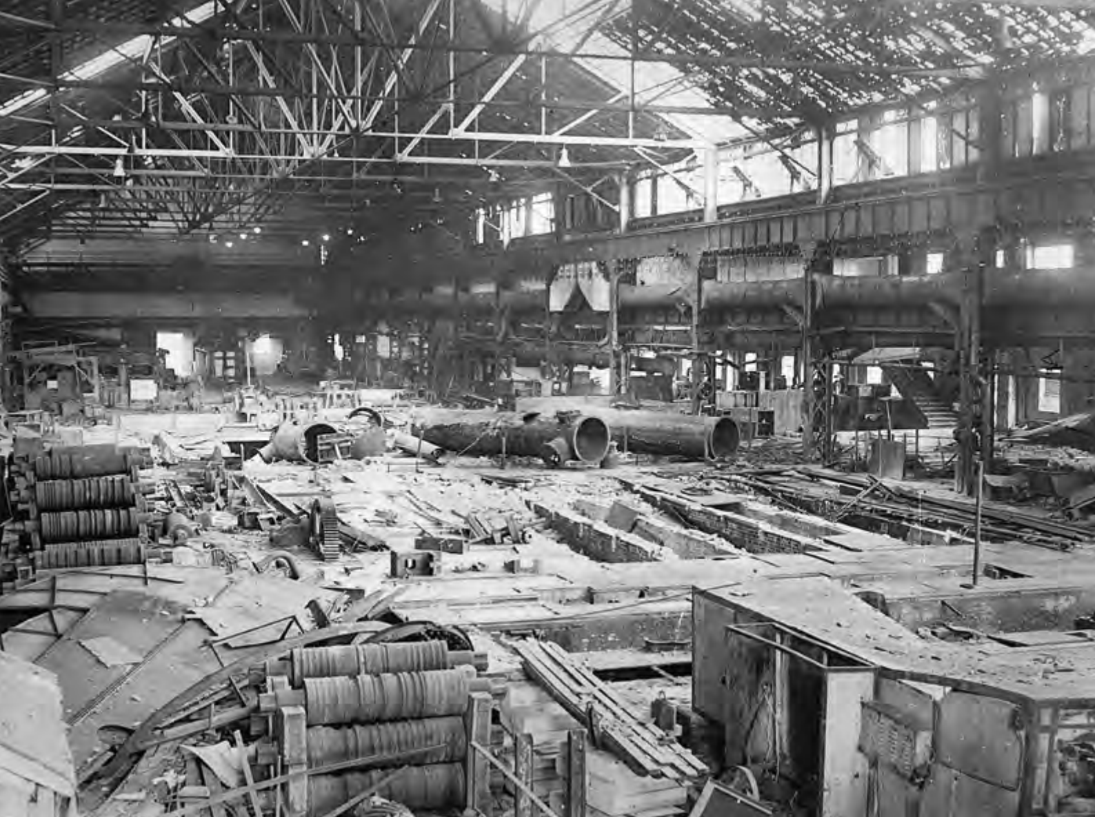
Hall complex of the metal plant in Berlin-Gartenfeld after the dismantling of the rolling mill, summer 1945
