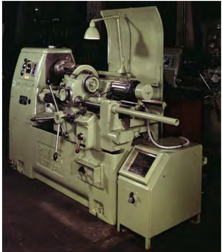
An automated lathe with SIMATIC components from the Pittler company, Langen, 1959
