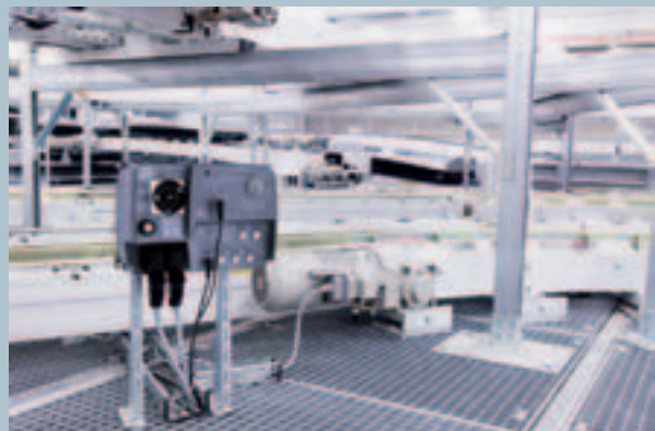
Innovation and testing center for airports
