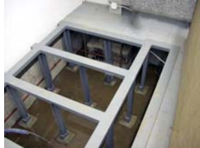
Fig. 22: Frame construction with longitudinal girders
