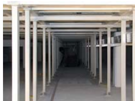
Fig. 23: Frame construction with longitudinal girders (cable basement)
