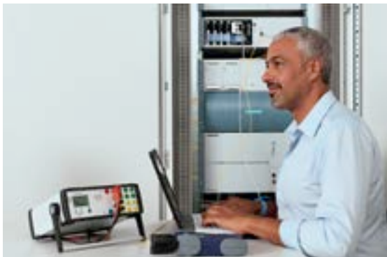
Commissioning of the SWT 3000
