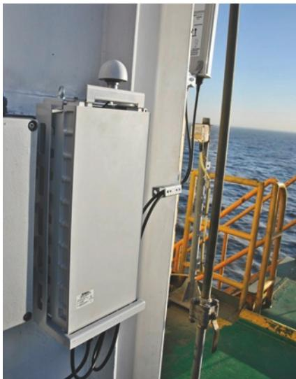
With the installation of Siemens wireless products, including RUGGEDCOM wireless terminals and RSN900NC switches, it was possible to integrate real-time data for units and transformers collected by platform power plants into the DMS. "In this case, after adding corresponding information for units and transformers to the DMS, Liaodong was able to monitor and manage units and transformers through the DMS system," adds Wenshuai.
