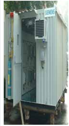
Compact Substation
