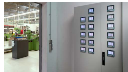
7KM PAC measuring devices in an Alpha distribution board from Siemens
