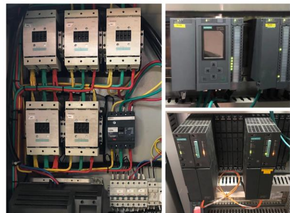
Siemens industrial products help intelligently control stage facilities during the complex movement sequences.
