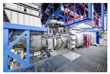
**Above:** With high exhaust heat and the ability to handle sudden load changes, the SGT-700 is ideal for simple cycle, combined cycle, cogeneration, and other heating applications.
