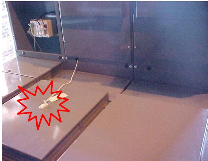
**Figure 14: Sensor placement for Switchgear cable termination chamber (External through Hole Detector)**
