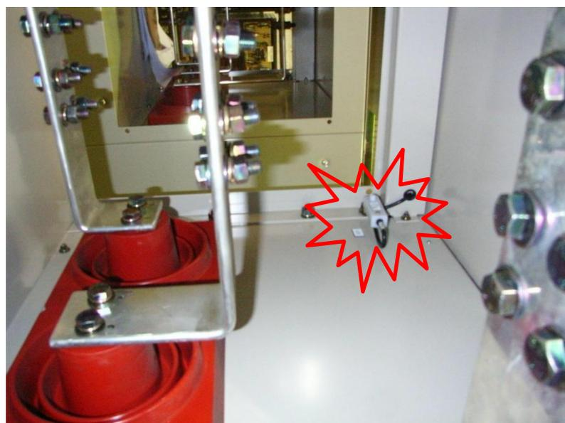
**Figure 8: Sensor placement inside busbar chamber**
