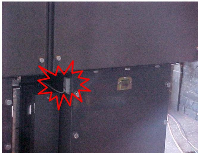
**Figure 12: Sensor placement for Switchgear cable termination chamber (External through Hole Detector)**
