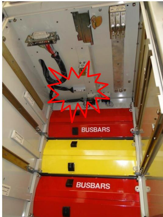
**Figure 7: Sensor placement inside CB racking chamber**
