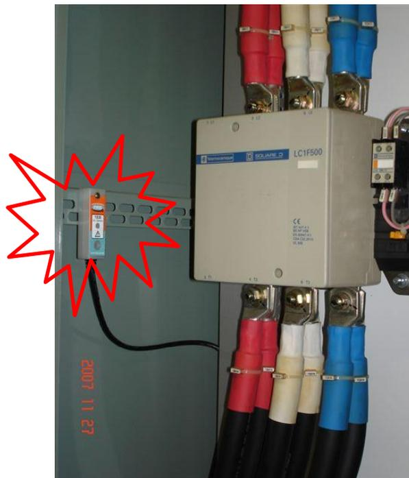
**Figure 11: Sensor placement near Low Voltage Contactor for a Variable Speed Drive**
