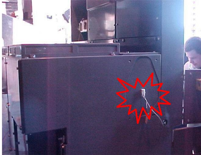
**Figure 13: Sensor placement for end of Bus chamber (External through Hole Detector)**
