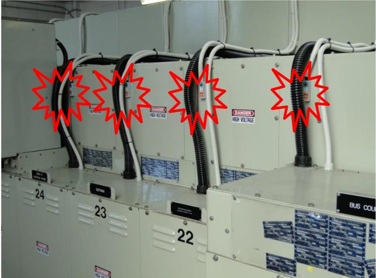
Figure 10: Sensor placement for switchgear Busbar coverage (External through Hole Detector)
