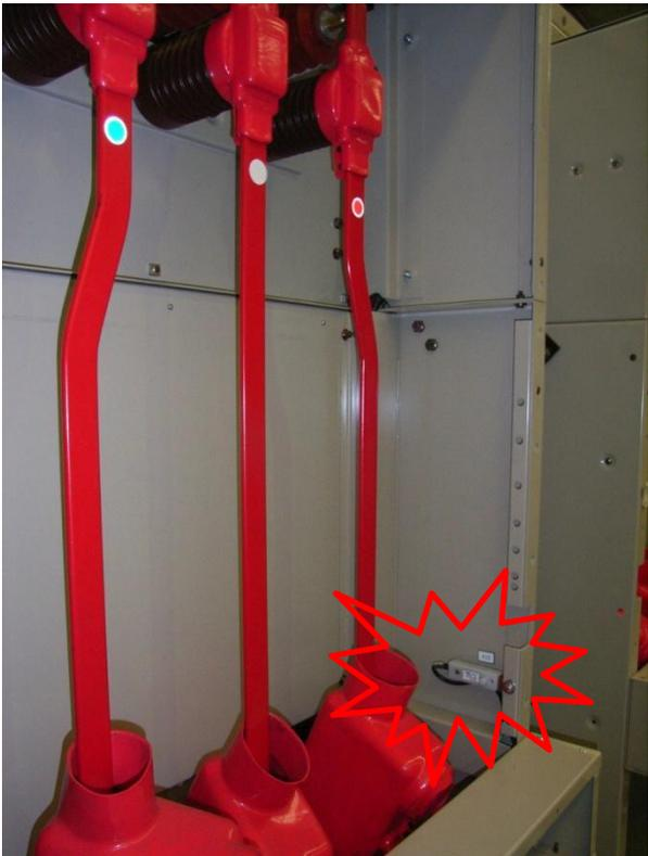
Figure 9: Sensor placement inside cable termination chamber
