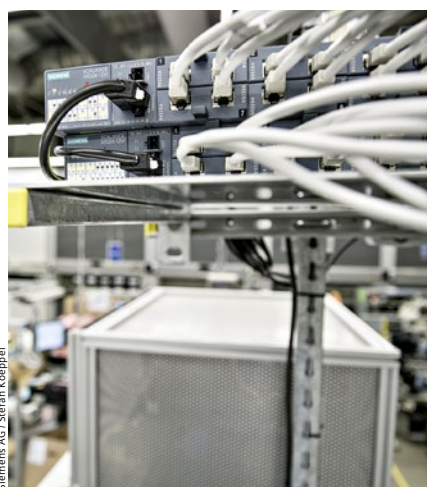
PCs and controls of the production lines and work stations are radially connected to the central data server via rack switches
