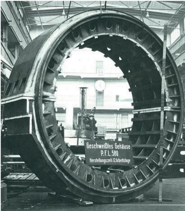
Figure 1: 1955, Siemens Motor with welded fixation of the stator core
