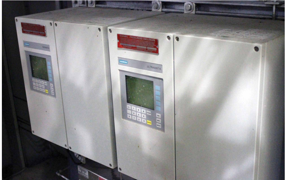
NCERC added a bank of OXYMAT and ULTRAMAT gas analyzers for measuring oxygen levels in the fermentation process.
