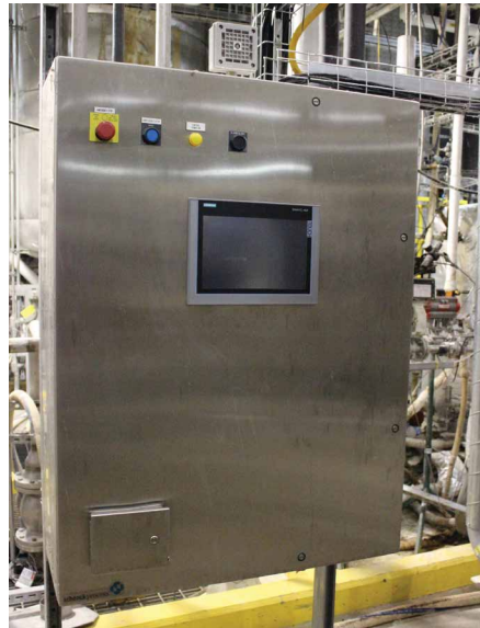
NCERC's installation includes SIMATIC PLCs.
