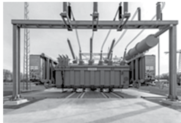
Ester filled Power Transformer
