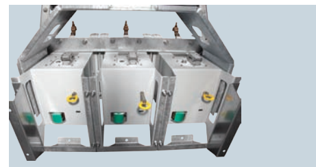
Figure 29: Bottom view of fully assemble triple-single recloser with phase B locked out
