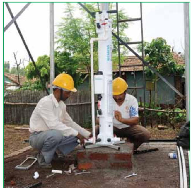
Siemens Ltd. has provided technology and support to make the remote, inhospitable hamlet of Amle into a model for the rest of the off-grid villages in India.
