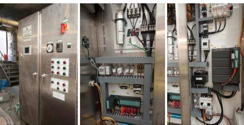
keep each pool's water moving at 30,000 gallons per minute. With its onboard CPU, the ET 200S distributed I/O nodes can offload computing tasks from the S7-300 master controller and permit much faster responses to time-critical signals.
