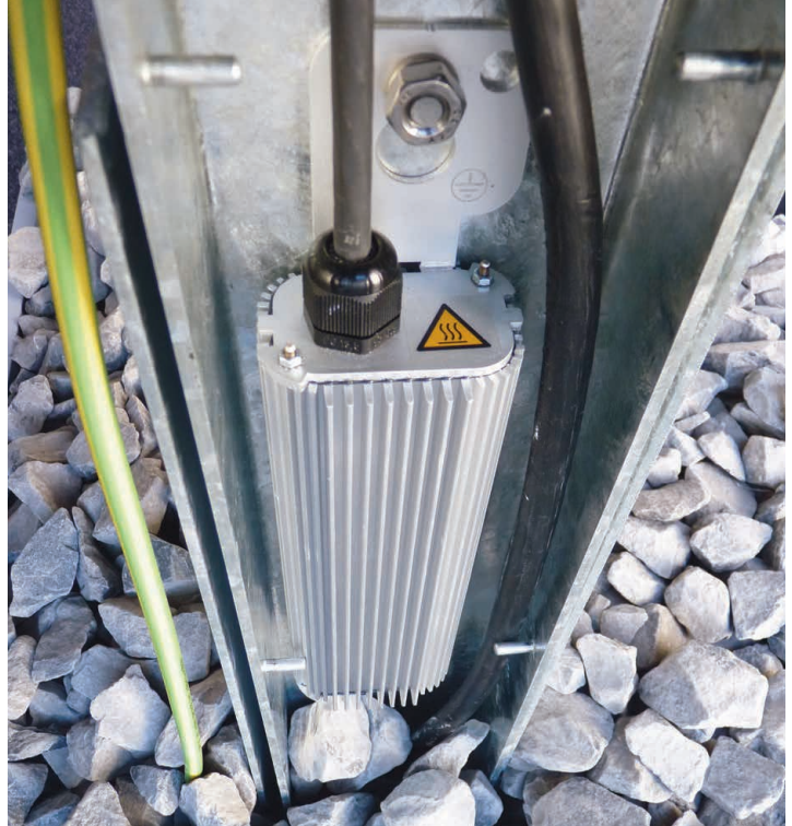
Resistor module integrated into the signal base
