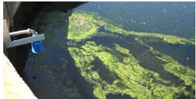
Figure 3.a.b.c. Effluent Discharge Basin V-Notch Weir for discharge flow measurement and Echomax Transducer for level measurement notice the algae build up
