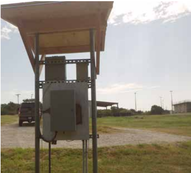
Figure 4.a.b HydroRanger 200 mounting stand and StoreIQ remote monitoring solution
