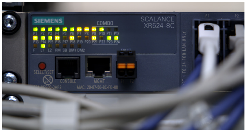
SCALANCE XR524-8C switch as the backbone of the production network
