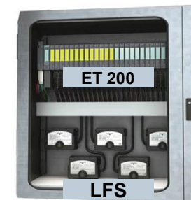
SIMATIC burner controller
