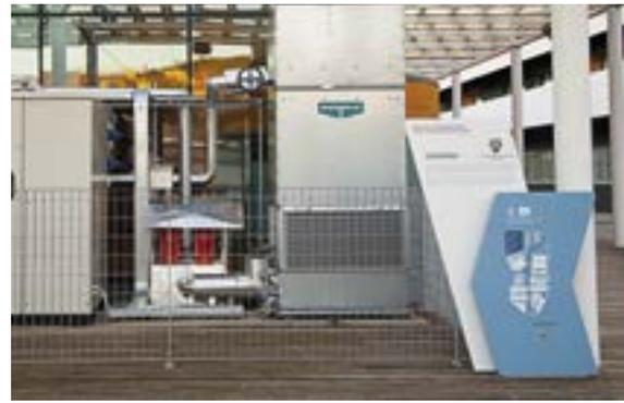
Absorption chiller that converts turbine waste heat into cooling energy
