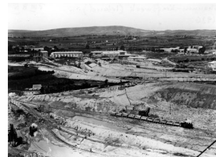
The powerhouse construction site in summer 1926
