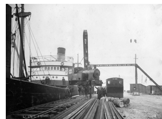
Unloading one of the 130 steam locomotives used during the construction work, 1926
