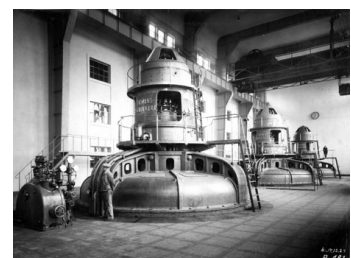
View of the generator hall, 1929
