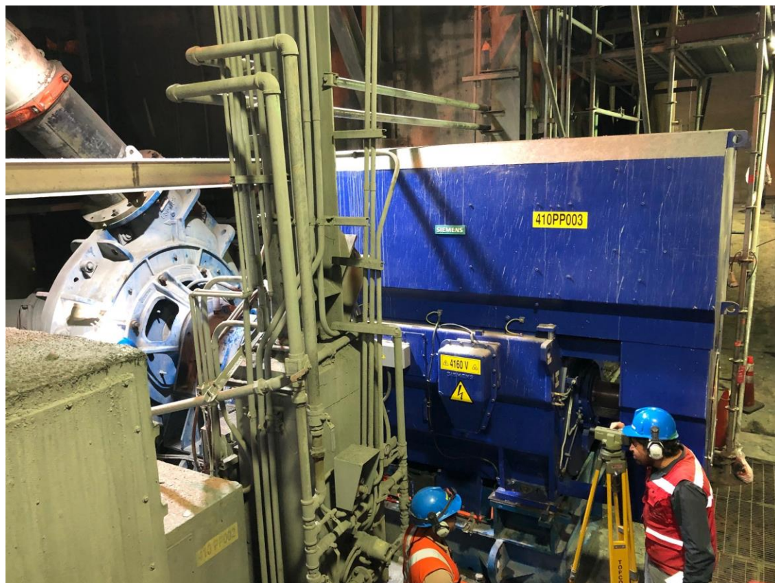
HV-M Motor 1560 kW 4.0 kV slurry pump application (gearbox)
