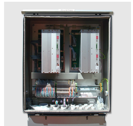
Two Trainguard LEU S21 in a trackside cabinet
