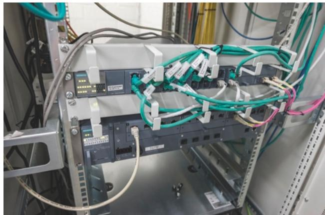
The SCALANCE X switches are installed in decentralized control cabinets.
