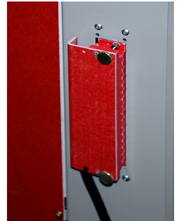
Figure 5: Split-plug jumper connected to circuit breaker
