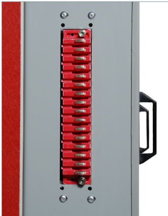
Figure 23: Secondary disconnect on the circuit breaker
