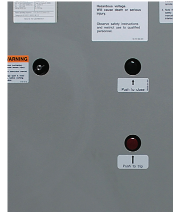
Figure 32: Trip-control pushbutton (lower button)
