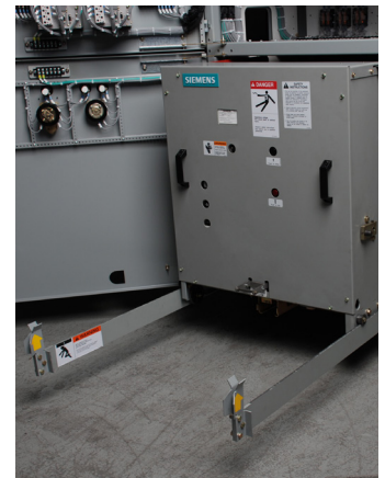
Figure 3: Use of extension rails for removal of circuit breaker not at floor level
