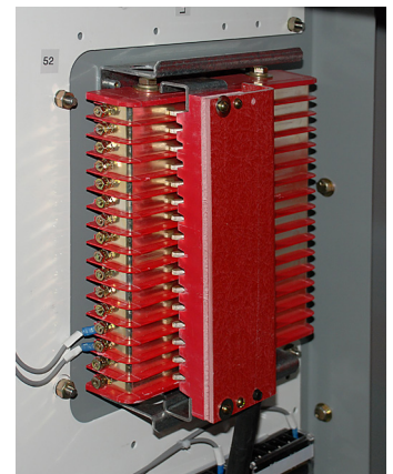
Figure 6: Split-plug jumper connected to switchgear
