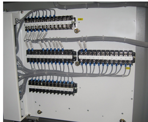
Figure 27: MOC (bottom) and TOC (top) switches and associated terminal blocks
