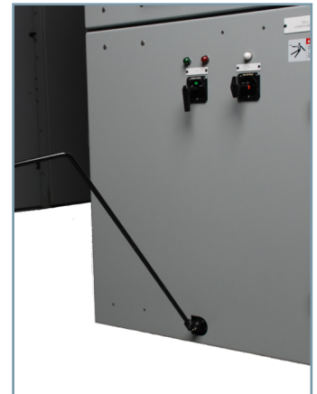
Figure 2: Type GMSG vacuum circuit breaker racking
