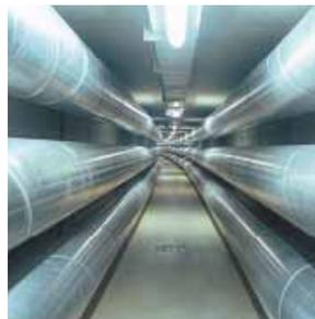
High efficiency from generation to consumption: In addition to our plant optimization technology, our gas-insulated power-line technology provides a high output transmission method which reduces transmission losses by two-thirds, compared to an overhead line.
