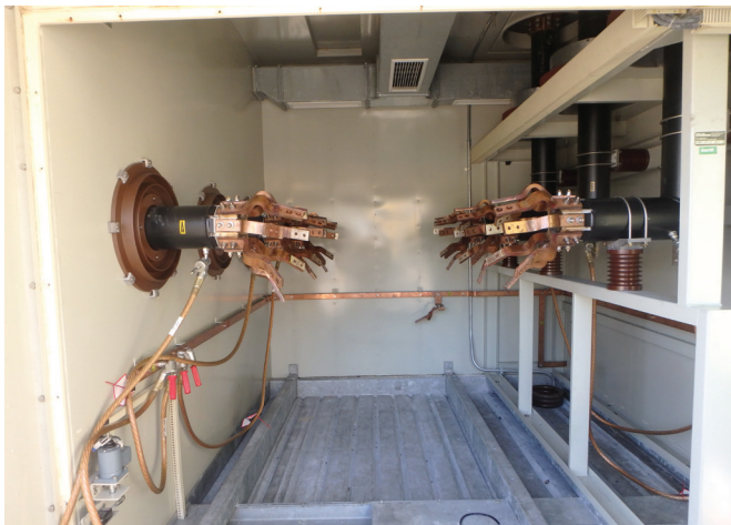
Figure 1. Visual progression of the replacement process, beginning with the existing SF 6 circuit breaker that is to be replaced and ending with the custom engineered Siemens vacuum replacement solution, installed directly into the existing gear requiring no modifications.
