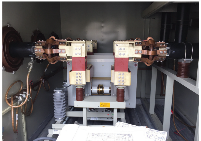
Figure 1. Visual progression of the replacement process, beginning with the existing SF 6 circuit breaker that is to be replaced and ending with the custom engineered Siemens vacuum replacement solution, installed directly into the existing gear requiring no modifications.
