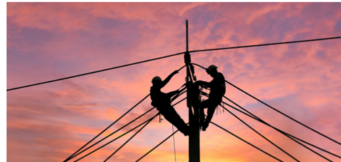
MV Outdoor Distribution Systems for a Reliable Grid
