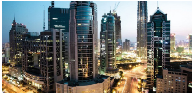
Financing for infrastructure
