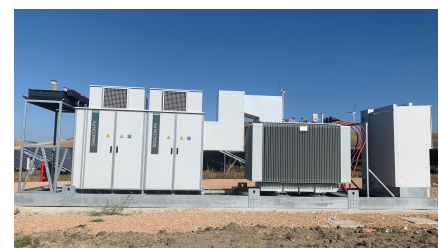
Troia energy site
