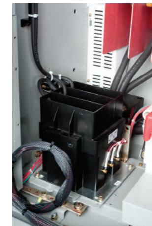
Figure 23: Voltage transformer arrangement in the feeder cell
