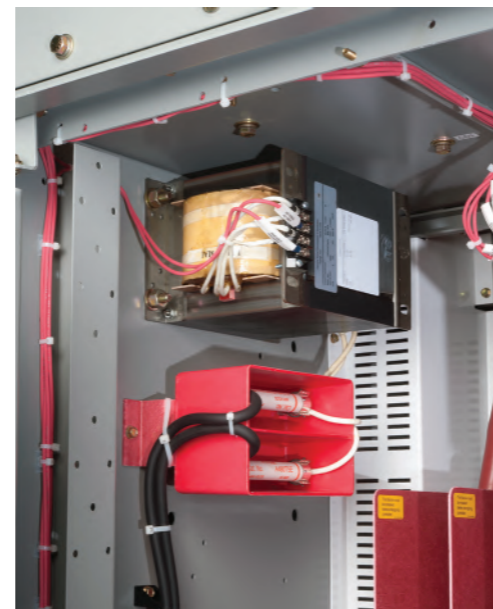
Figure 22: Control power transformer mounted in the cell
