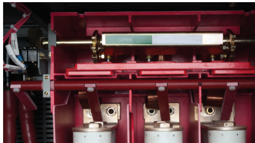
Figure 14: Blown fuse trip mechanism (optional)
