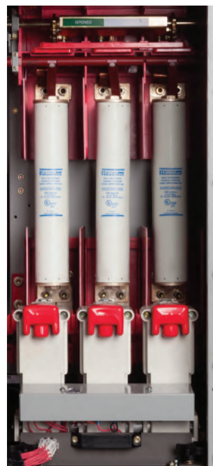
Figure 32: Power fuses
