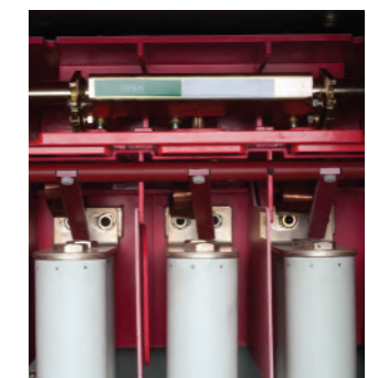
Figure 9: Isolating switch (shown in OPEN position)
