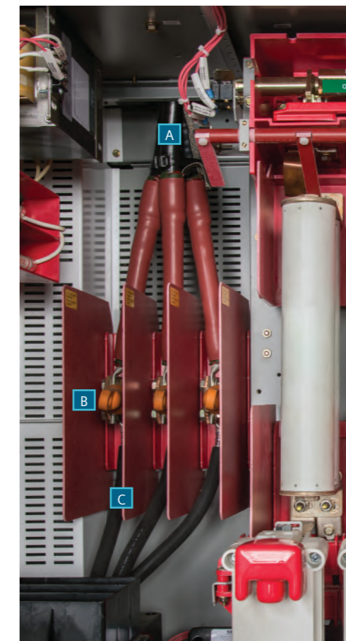
Figure 26: Typical outgoing connections
