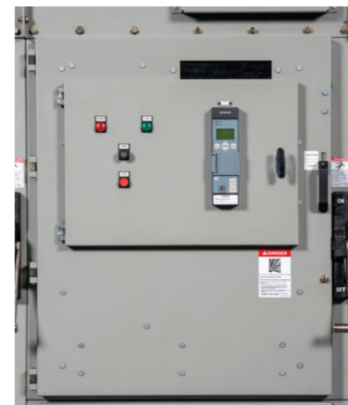
Figure 8: Low-voltage and medium-voltage compartment doors (400 A)
