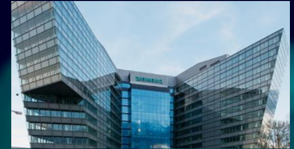
Microgrids for Siemens, e.g. in Vienna, Milan, Midrand
