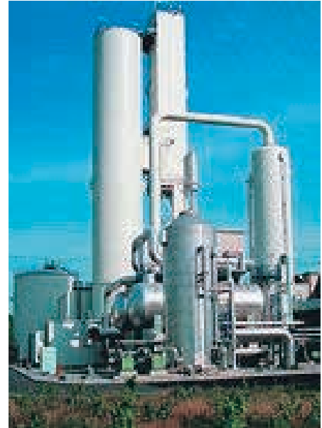
Fig. 2: Typical air separation plant
