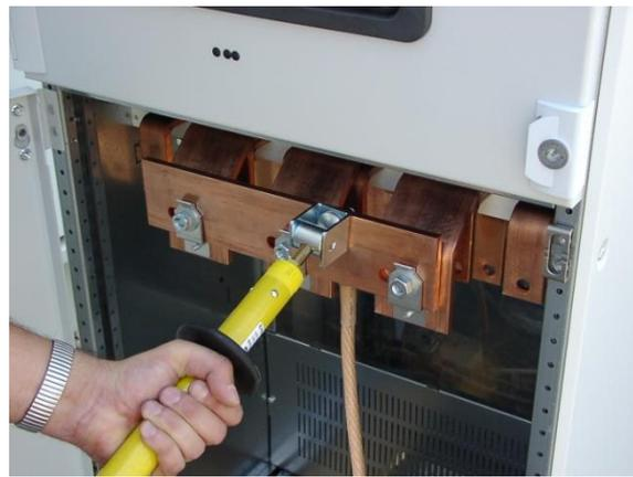
Fig. 11: Shift the bar downward to the end position, then (only with breaker size 2 or 3) sideward to the end position.
