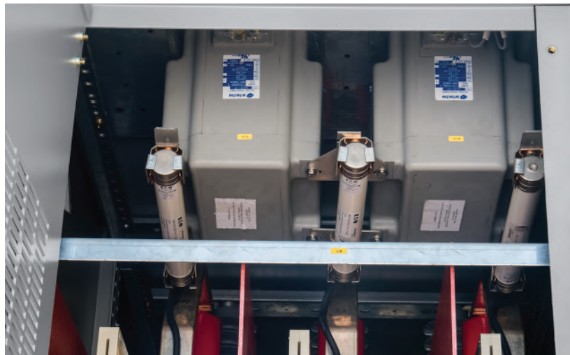
Voltage transformers located above the switch
