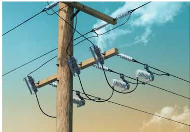
open for a pre-determined time (dead time). Then the Fusesaver closes again and remains closed. Depending on the type of fault, there are distinct effects on the feeder.
