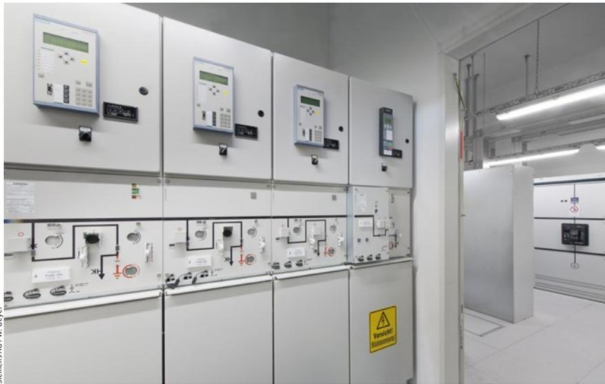
From the transfer station, two independent supply paths lead to two 8DHJ medium-voltage switchgear assemblies separated by a firewall
