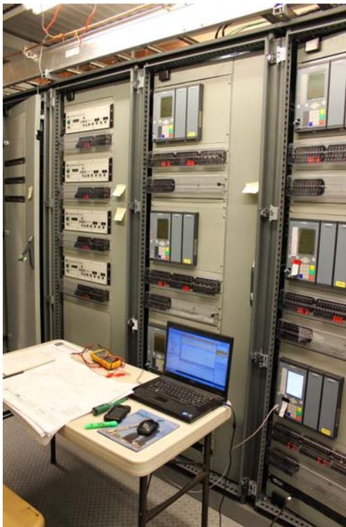
Testing of New Control Enclosure Relays
