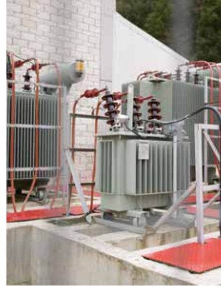
Oil-immersed distribution transformers
