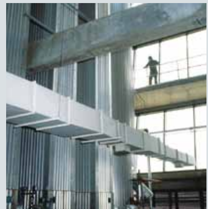
The Passaic Valley, New Jersey, municipal treatment plant uses twelve Zimpro® wet air oxidation systems for municipal sludge treatment, each with a capacity of over 60 m 3 per hour.
