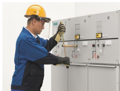
Figure 1: Working on live equipment
